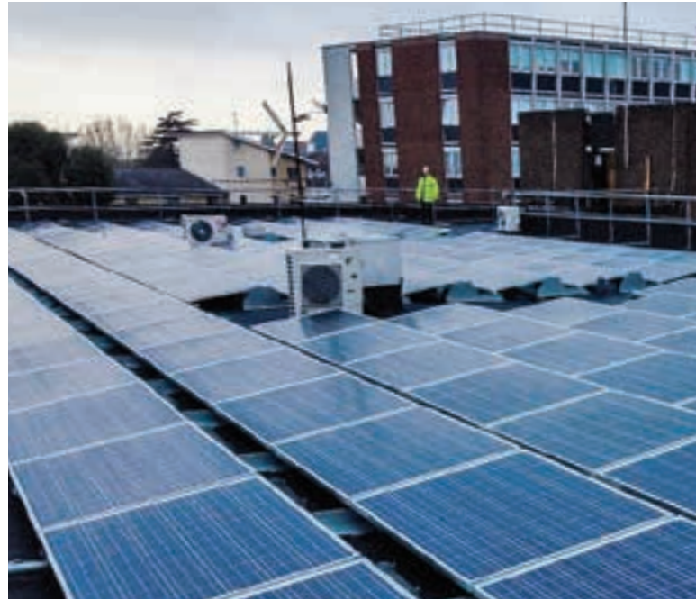
This 50kW(p) solar array was installed on Chelmsford Council's main offices in just one week.
